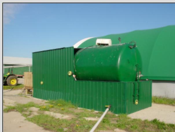
Fig. 3 – Anaerobic digester – main digestion tank is at right end
