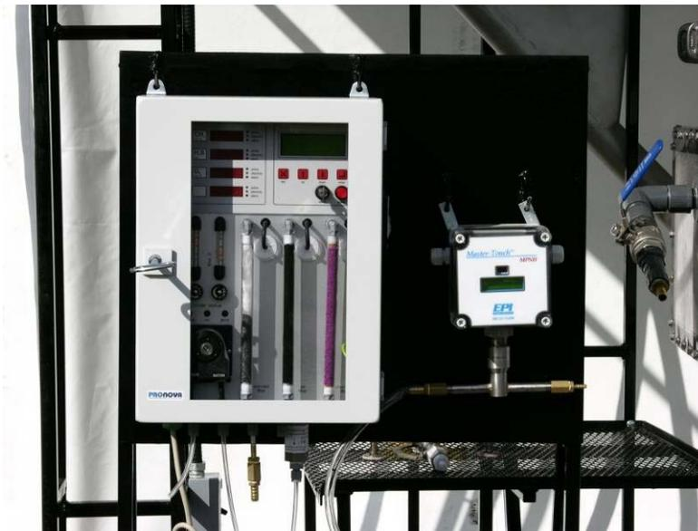
**Figure 7 Equipment for measuring gas flow rate and volume and for analysis of methane, oxygen and hydrogen sulfide**
