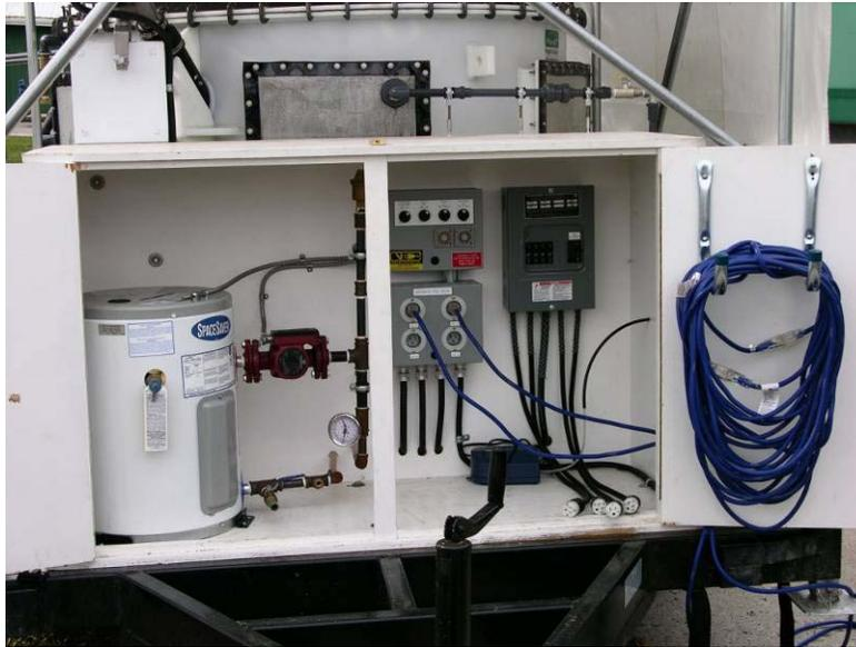
**Figure 6 End compartment housing the water heater and electrical panel - wired for 115 and 230 V**
