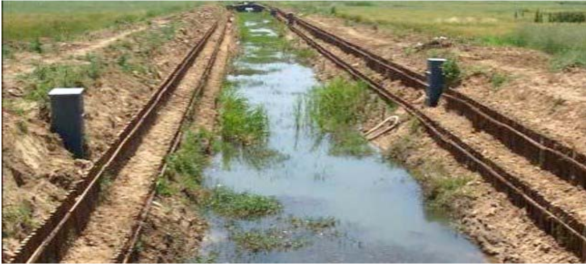
Figure 5. Photo of the ditch wetland at Yaxi town WRSIS site
