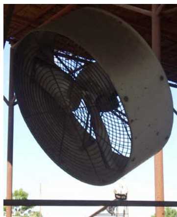
Figure A.4. Modified fog cooling system to micro-sprinkler and fan cooling system.
