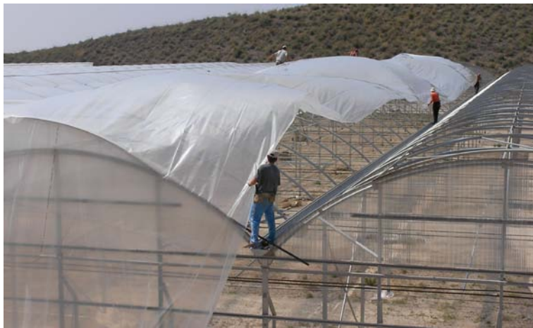
Figure 2: actual methodology: spread out the plastic film
