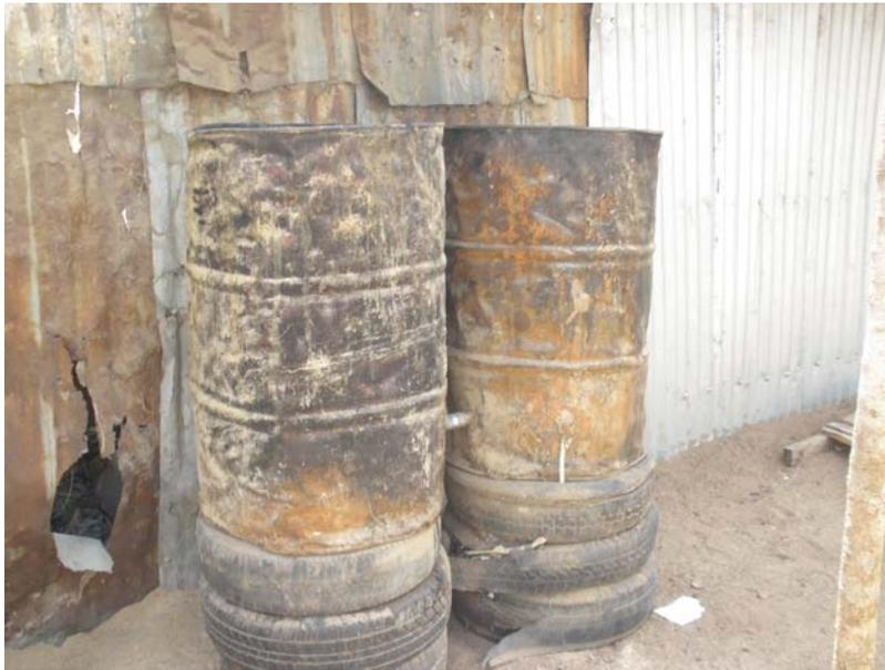
Figure 4. Diesel engine cooling system consist of two barrels at atmospheric pressure
