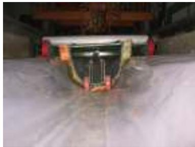
Fig. 6. The process of paving geomembrane on the U-shape canal
